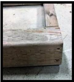
Make the frame of the trap door from the 2x4 and 4x4 as seen in the picture by cutting (using the circular saw) so that the 4x4s are used for the the wheel to wheel width and the 2x4 is used for the length. Screw them together by putting 2 screws in each end of the 4"x4".
